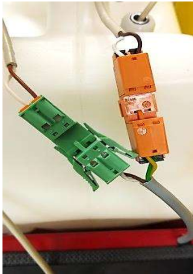
Fig. 10.3 Properly connected float switches
